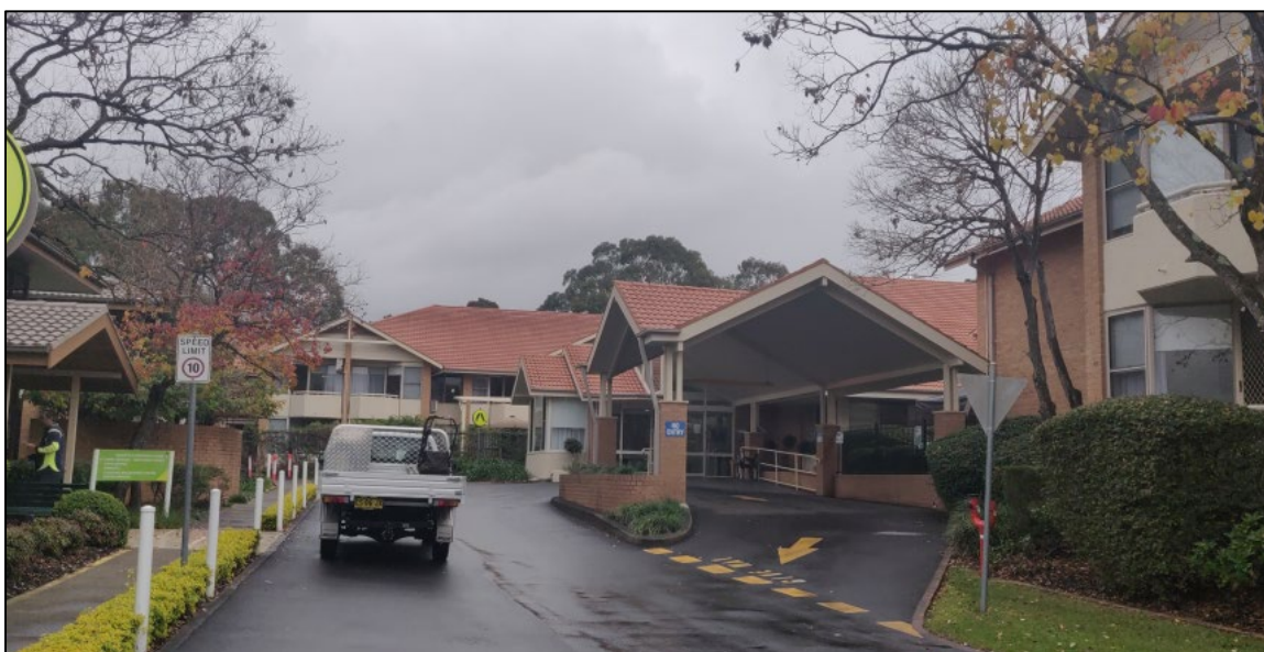
Figure 6: BaptistCare buildings to the west
